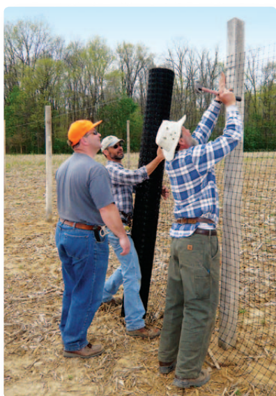
A group of volunteers install a section of the Banks Hardwoods sponsored deer fence.
